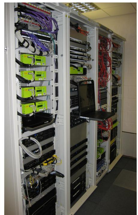
*iTrinegy's NE-ONE Professional and NE-ONE Enterprise Network Emulators (green appliances) are an integral part of LSRC's test set-up*
